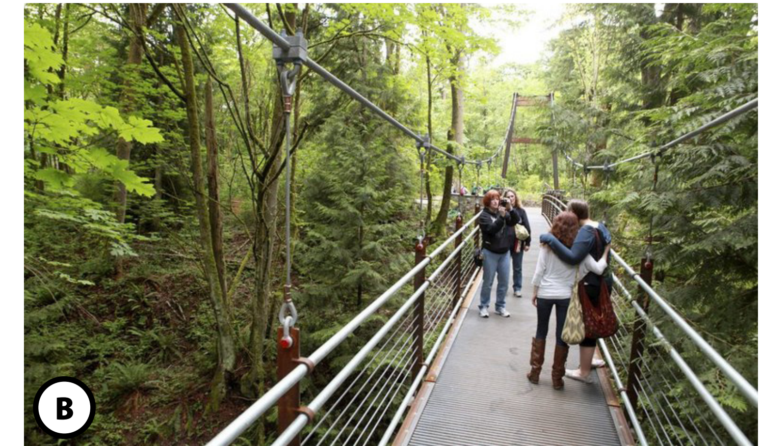
B Ravine Bridge Connecting Quarries
