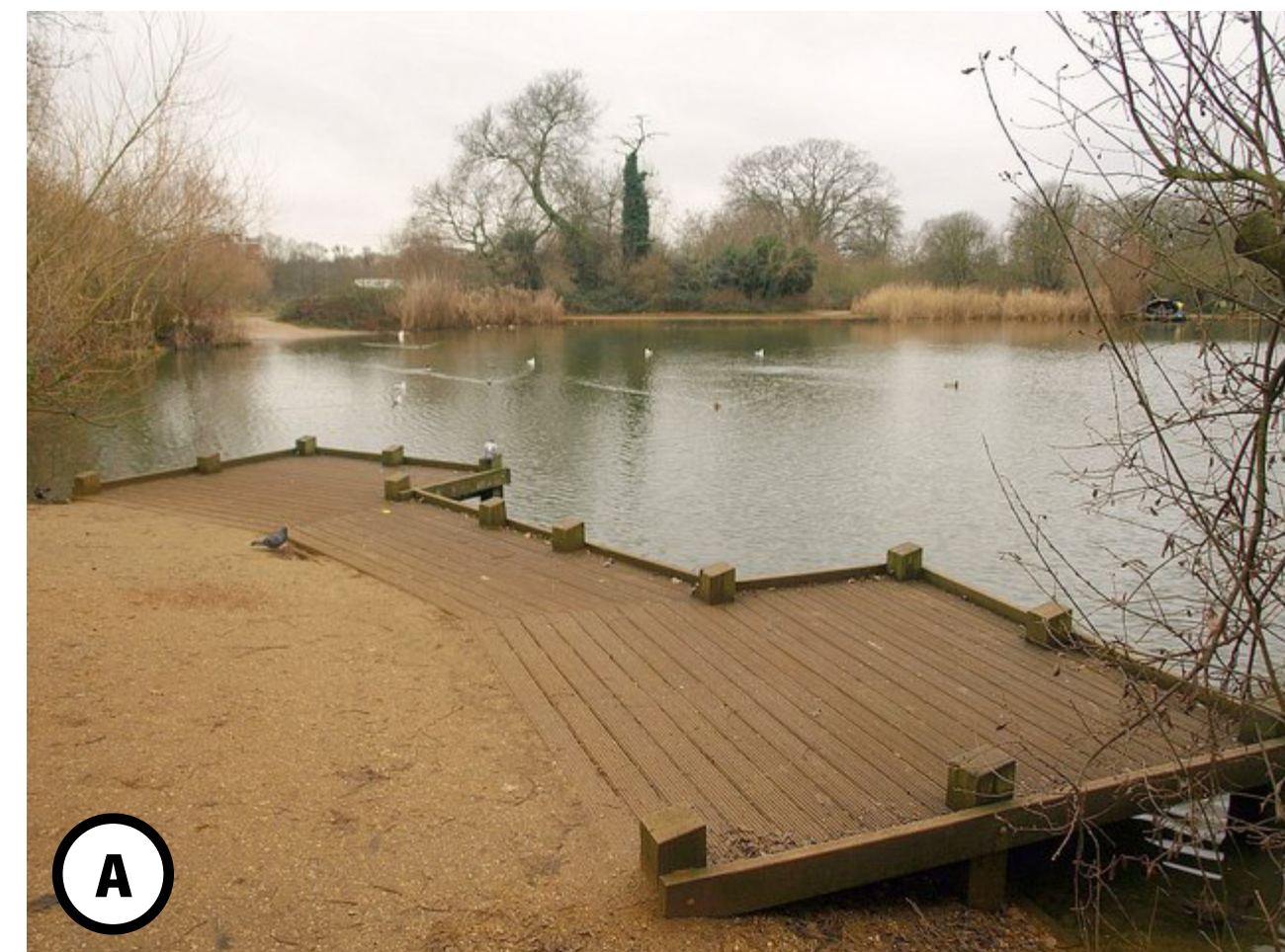
A Shore Fishing Pier/Platform
