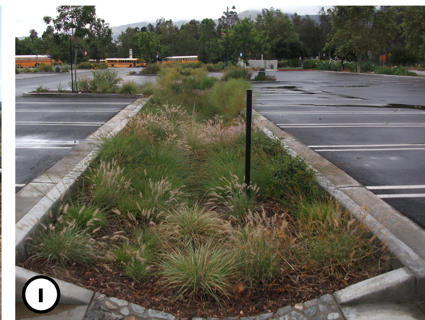
I Stormwater/Parking Lot Greening
