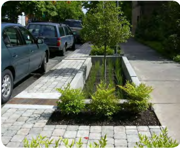
Stormwater planters are an attractive and beneficial way of collecting stormwater runoff
