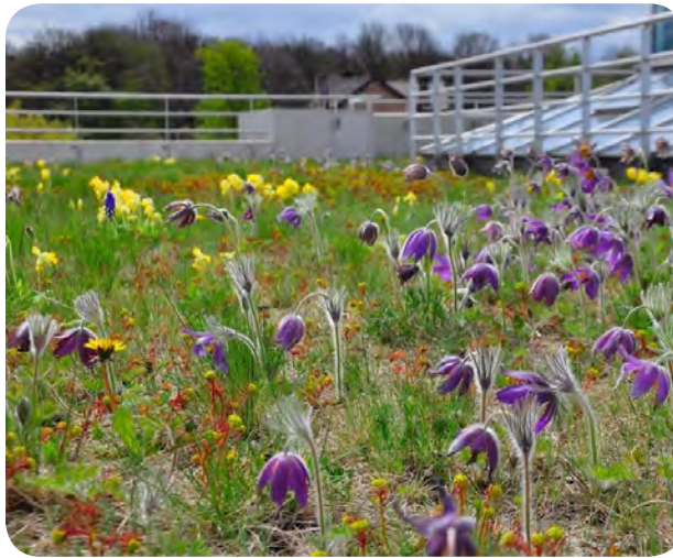
Green roofs can reduce stormwater runoff and the urban heat-island effect
