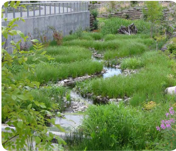
Raingardens and bioretention basins for stormwater management
