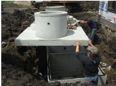
FIGURE 3 GRAVITY GREASE INTERCEPTOR
