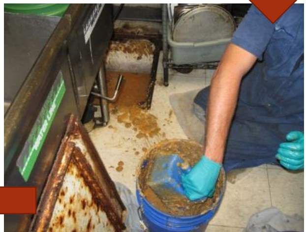
Remove solids from the bottom
