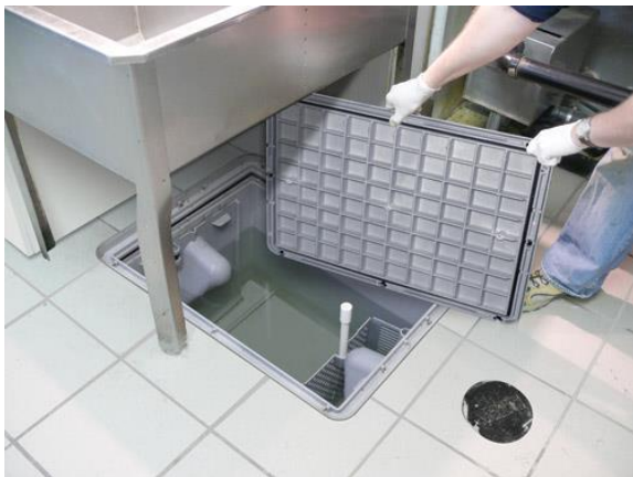
FIGURE 4 HYDROMECHANICAL GREASE INTERCEPTOR
