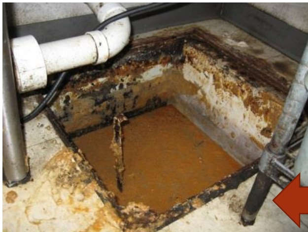
Scrape sides and inspect the interceptor
