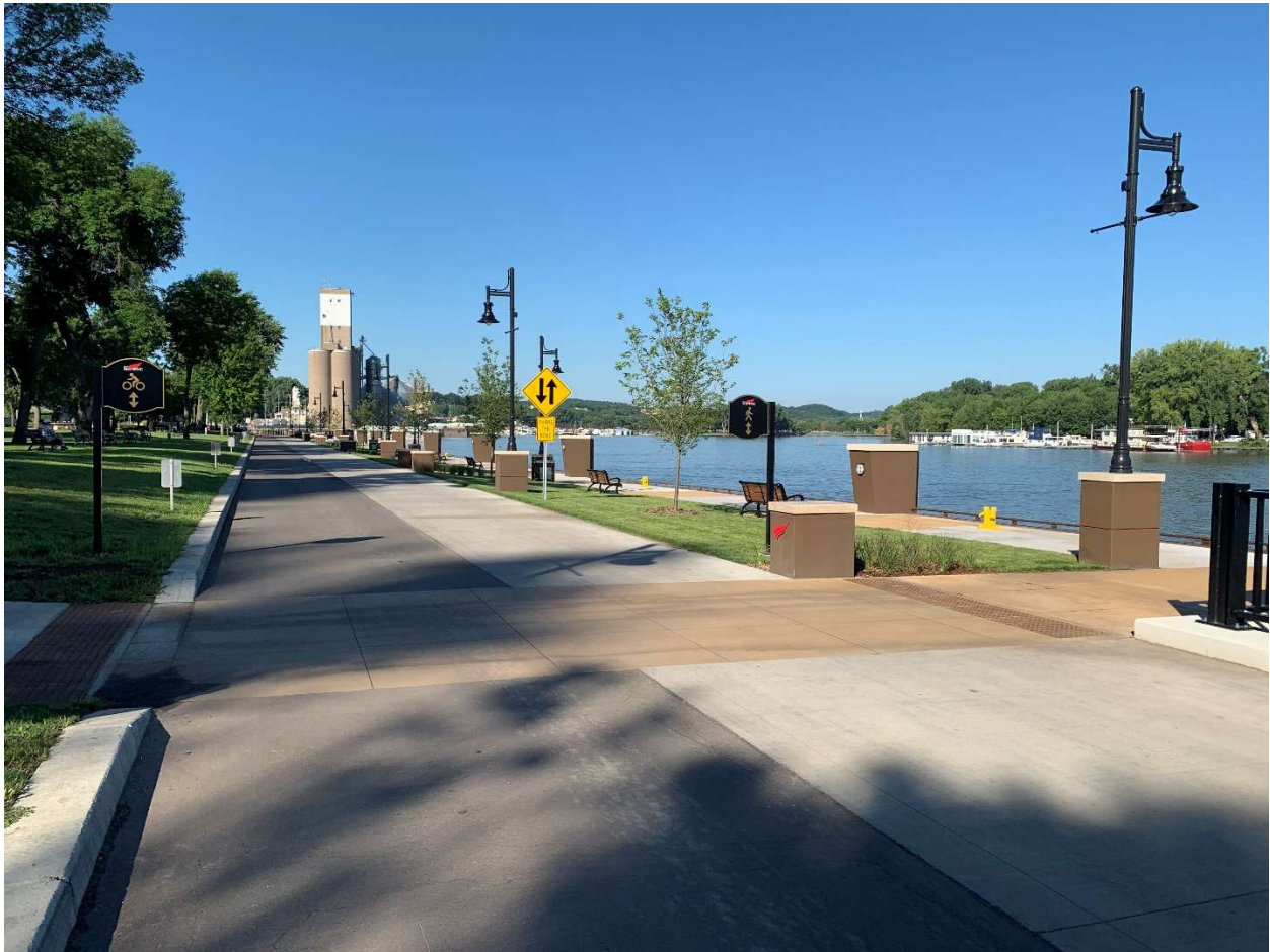
Photo courtesy of Kimley-Horn, Inc., CIP Project - Levee Park Dockage and Riverfront Trail 2020
