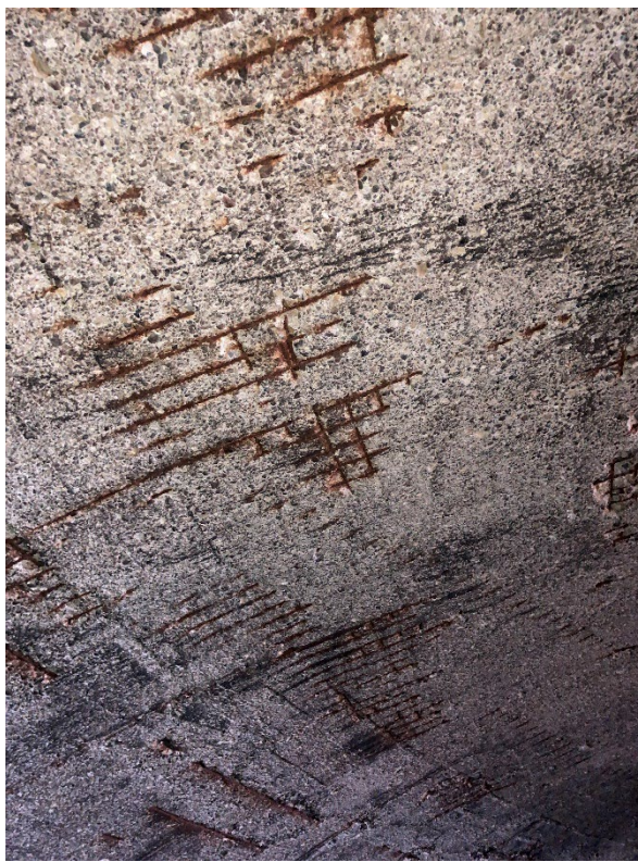
(Left) Small chunks of concrete from the dome have fallen onto the trickling filter media. (Right) Welded mesh and #4 ring rebar has lost concrete cover.
