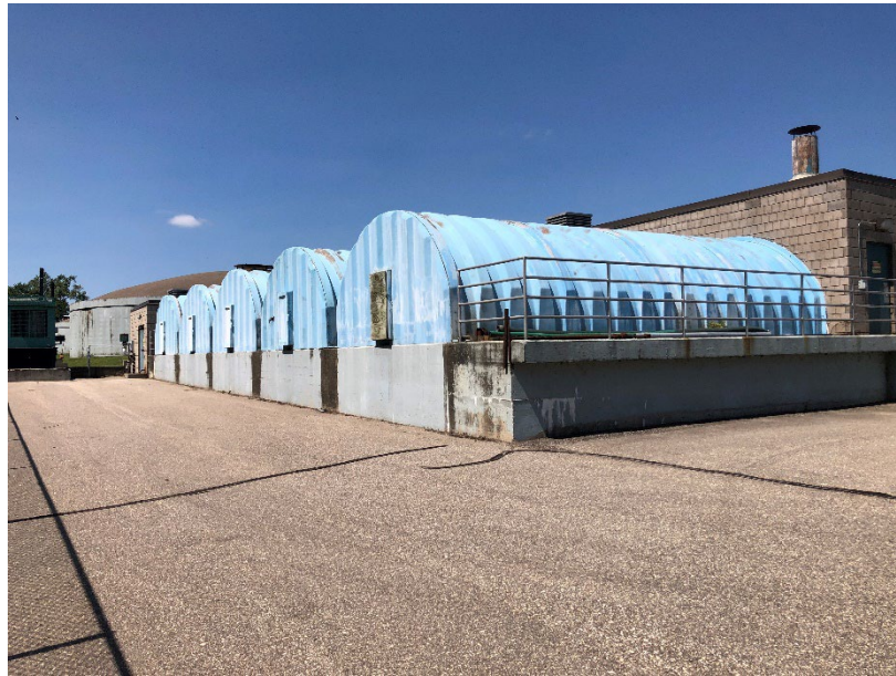
Figure 8 – Rotating Biological Contactor Exterior
