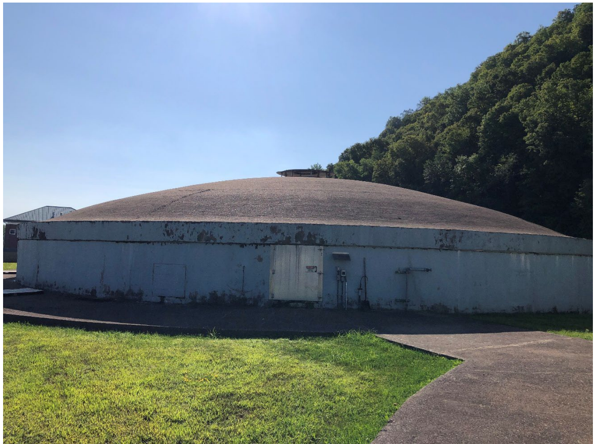
Figure 7 – Trickling Filter Exterior
