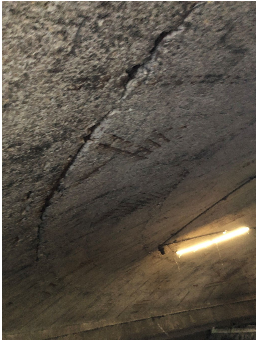
Figure 6 – Trickling Filter Roof Interior
