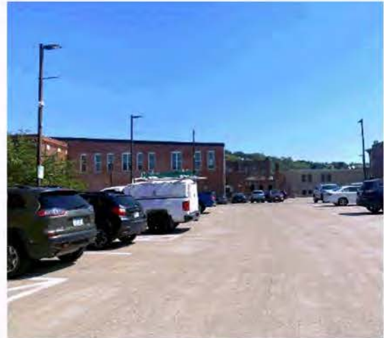
Top floor of the Studebaker Ramp in Red Wing.
