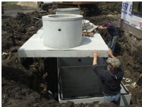
FIGURE 3 GRAVITY GREASE INTERCEPTOR
