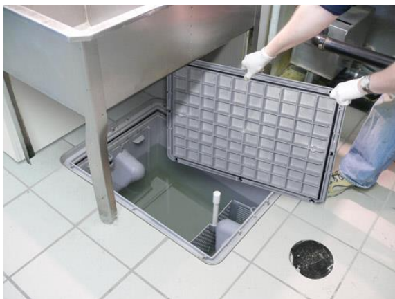
FIGURE 4 HYDROMECHANICAL GREASE INTERCEPTOR
