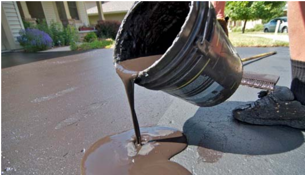
Pouring seal coating on a driveway.
